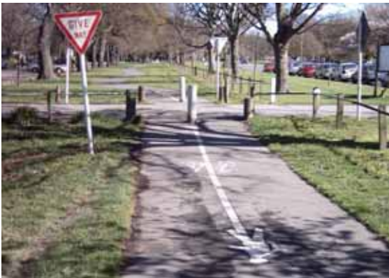
Figure 6: Busy path giving way to minor access road – South Hagley Park
