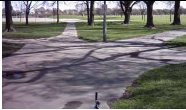
Figure 8: A five-leg path junction with no clear indication of right of way
