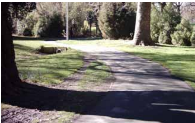
Figure 1: Sharp curves combined with poor sight distance
