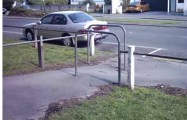
Figure 24: Unacceptable access for people in wheel chairs as well as cyclists
