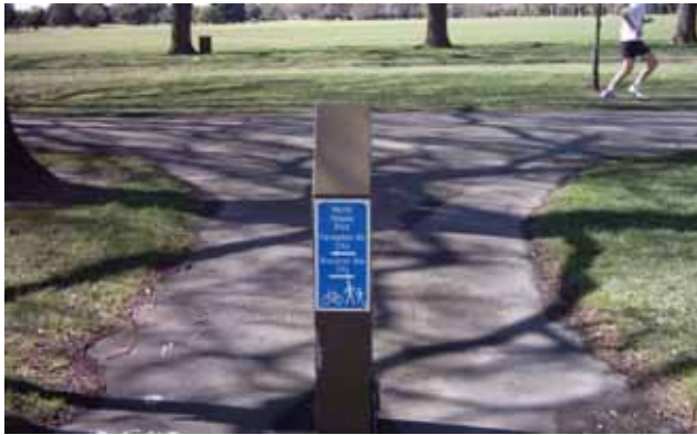
Figure 10: Good directional signposting, but far too small to be read while moving at normal cycling speed
