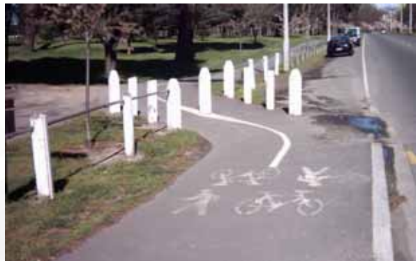
Figure 22: Access of reasonable standard
